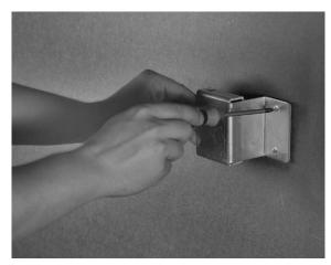
Drill 2 holes, put wall anchors in pre-drilled holes and then screw bracket into wall
